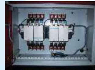
4P Contactor Switch
